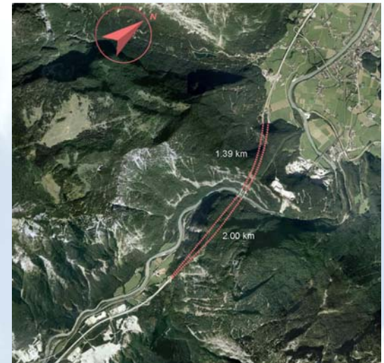
Fig. 1: Aerial view of the investigation site, a highway tunnel system (Ofenauer Tunnel 1.4 km, Hiefler Tunnel 2.0 km). Modified after Google Earth.
